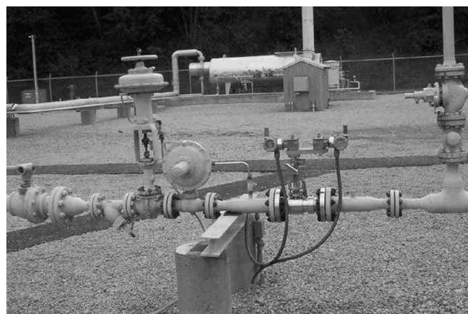
Application: 3" Sch 40 Natural Gas Operating Pressure/Temperature: 80 psig/70° F Max/Min Flow Rate: 60,000 SCFH/1,000 SCFH Flow Turndown: 60:1
